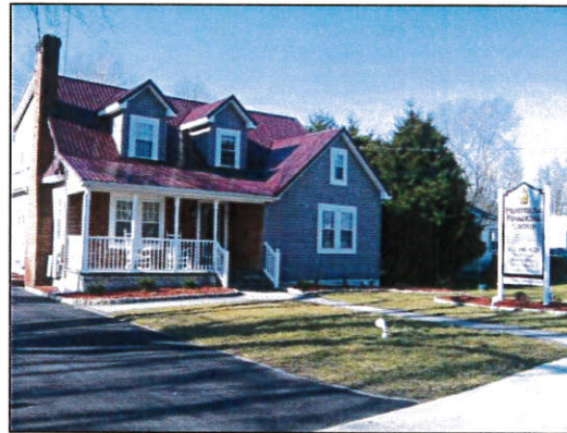
A building with access to the entrance from the driveway as well as sidewalk.
